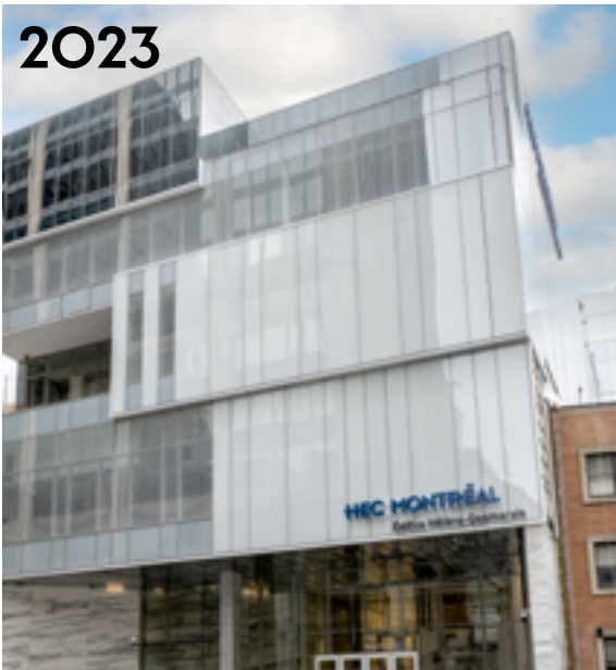
Hélène Desmarais Building
